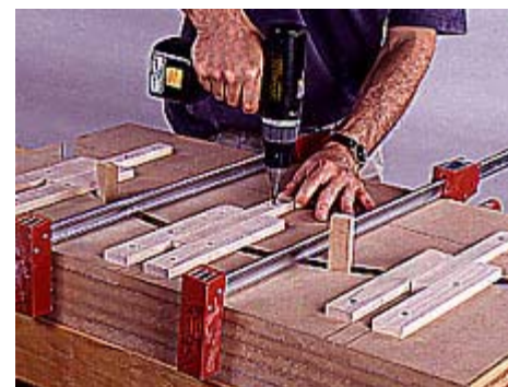
3 Use 3/4-in.-thick spacers between the bending form pieces. Clamp the form pieces together and fasten alignment strips.
