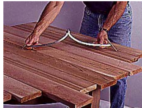
11 Space the boards equally, and screw them to the cross rail. Draw the outline of the top on the boards.
